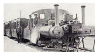
2 engines, side by side, straddle a single rail
